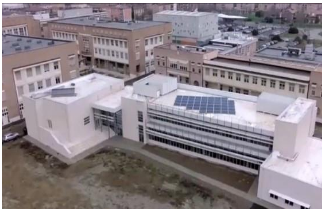
Figure 1: Flat roof with cool white waterproofing film [16].
